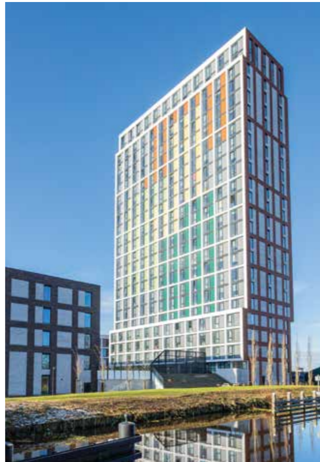
Zernike Tower – Groningen
