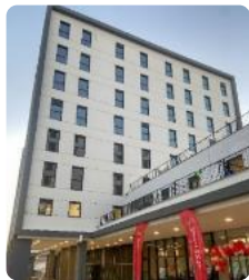
Lumiar, PT (498 units)
