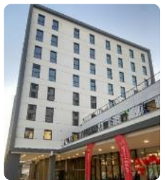
Lumiar, PT (498 units)
