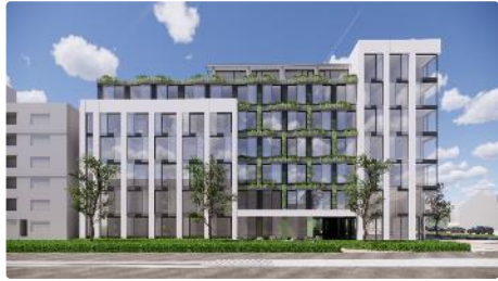
Boschdijk, NL (c.150 of 240 units) (delivery in Q1 2024)
